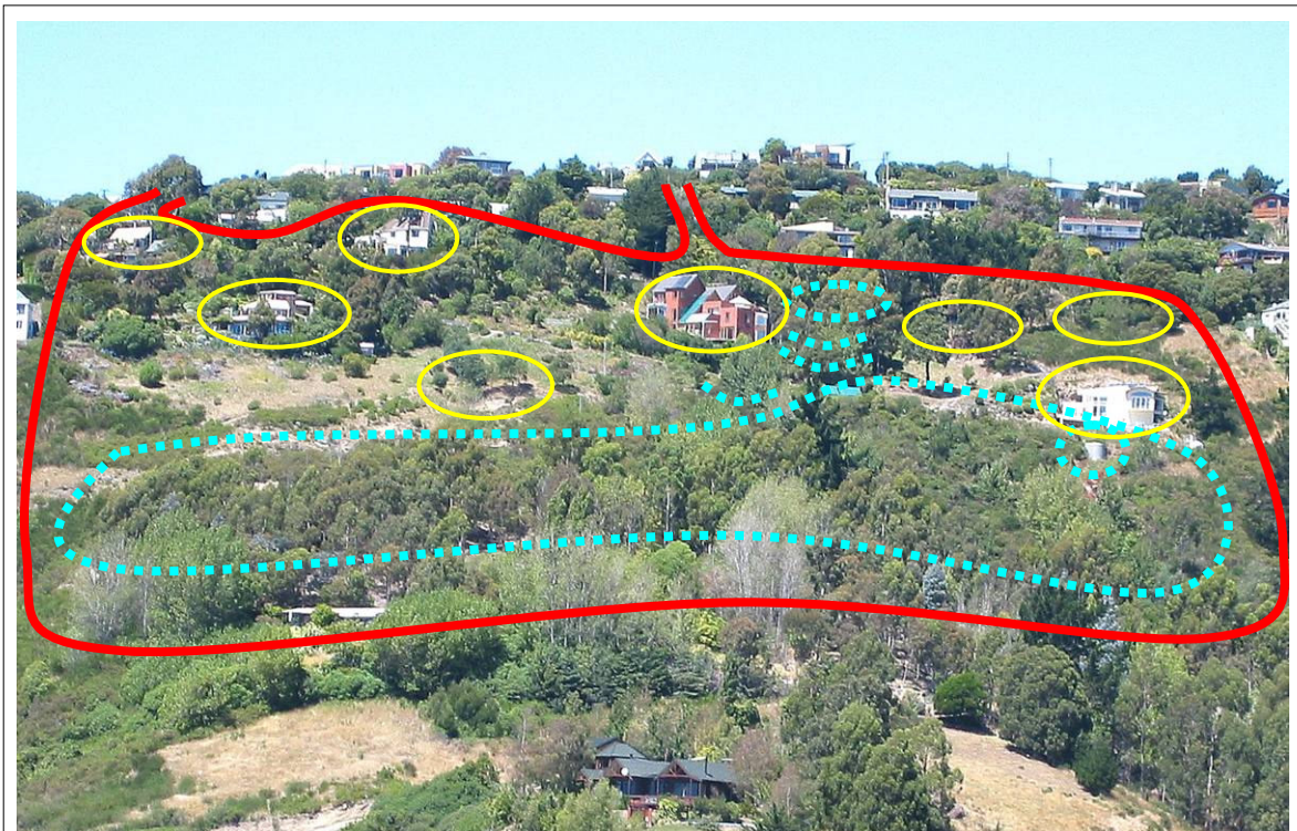
The photo shows in red the development boundaries, in blue the storm water containment and distribution system and in yellow the existing and planned properties on the Kakariki site.
