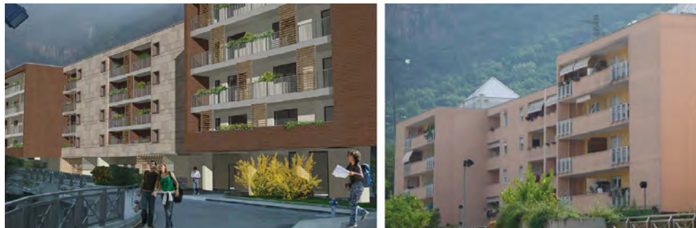
Figure 30 - (Left) North Building: render of the project. (Image: © Studio Mellano & ARCH+MORE); (Right) North Building: current status. (Photo: © Eurac Research)
