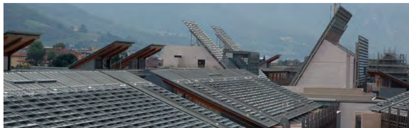
Figure 37 - System geometry: view of the PV systems integrated in the roofs from the terrace of the MuSe (Photo: © Silvia Croce).
