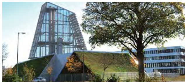
Figure 34 - Chimney of the heating plant of Freiham, including PV modules. (Photo: © Stadtwerke München)
