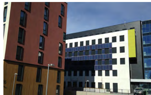
Figure 18 - A view of PV system installed on the South façade that resulted partly covered by the shadowing. (Photo: © Carmel Lindkvist)
