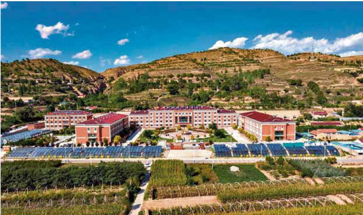
Solar combi-system consisting of flat plate collectors and a heat pump for space heating at a nursing home in Guyuan County, Ningxia
