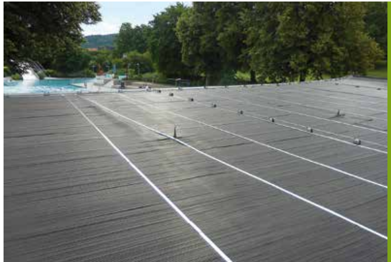
Solar system for outdoor pool Obersulm, Germany Photo: AST Eis- und Solartechnik GmbH, Austria
