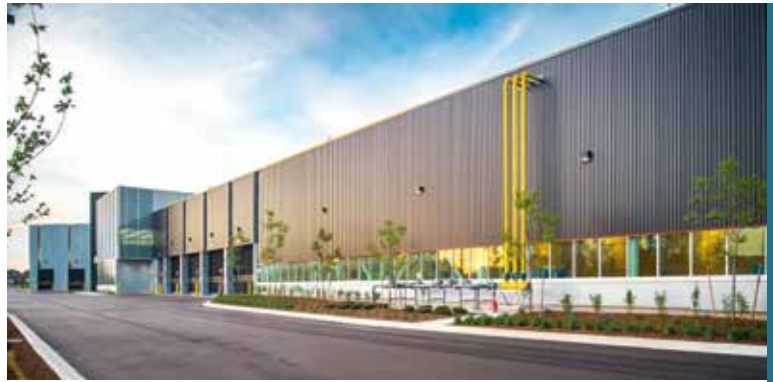
Toronto Transit Commission (TTC) McNicoll Bus Garage; Toronto, Canada
