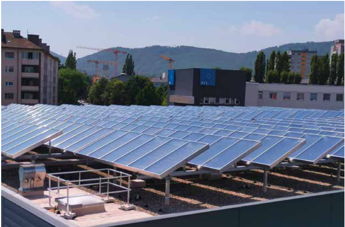
3,500 m 2 flat plate solar collectors supply heat to drive a 660 kW absorption chiller at the company AVL in Graz, Austria
