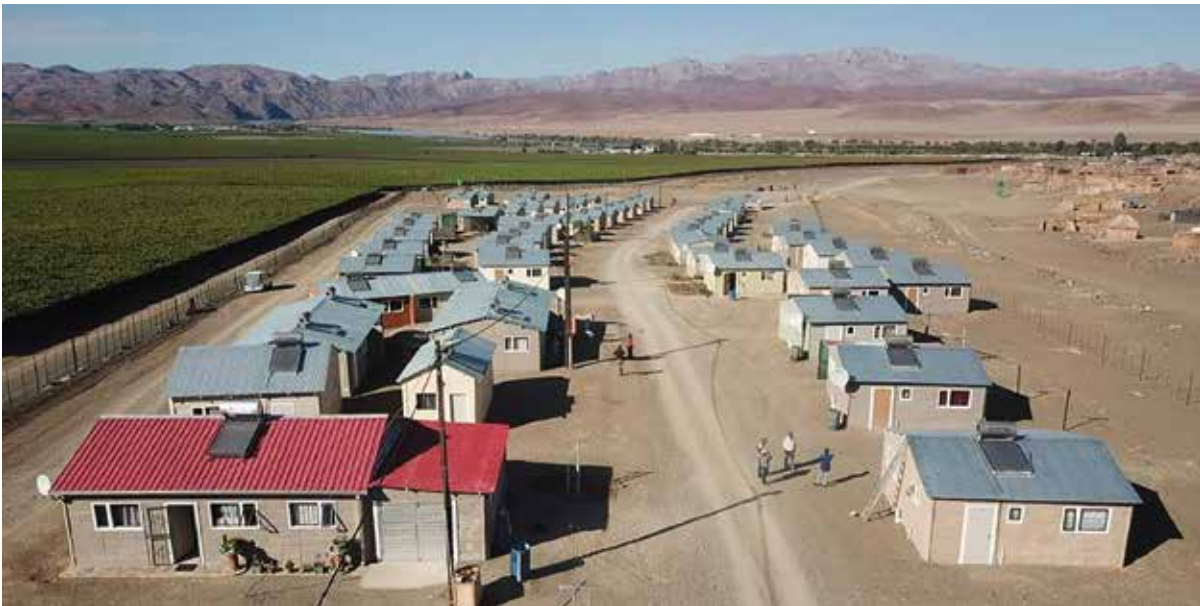
Aussenkehr, low-cost social housing project, Namibia
