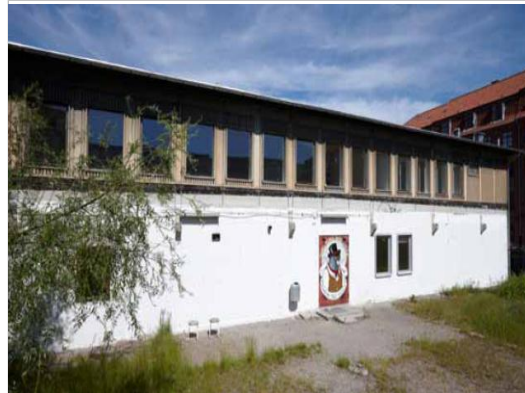
Façade facing garden - Before renovation
