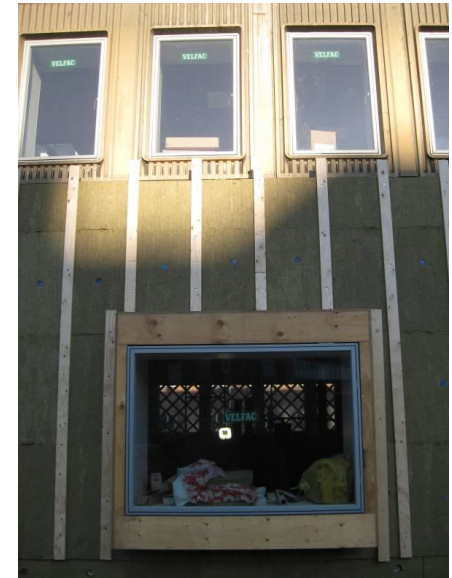
The ground floor of the back façade was insulated from the outside.
