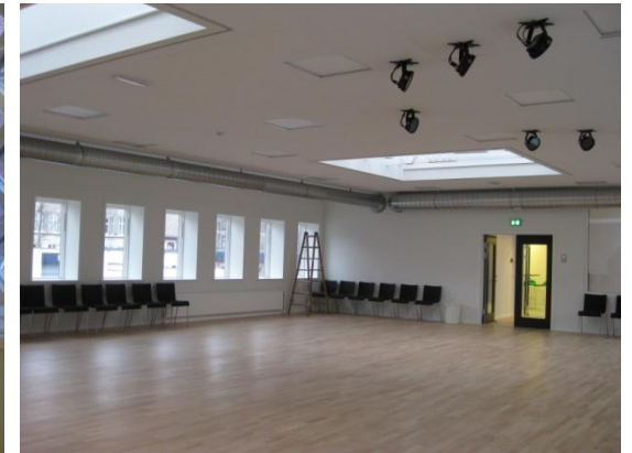
Daylighting and natural ventilation via roof windows.
