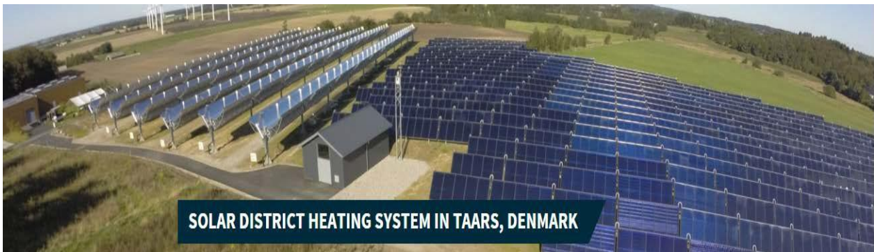
Fig. 2 The hybrid solar collector field of the Taars plant (Source: Aalborg CSP A/S).
