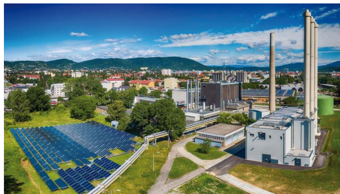
Figure 1: Collector array of plant Fernheizwerk . Source: Picfly.at Thomas Eberhard
