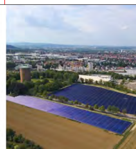
▲ Example of solar district heating plant in Ludwigsburg, Germany. Source: Guido Bröer
