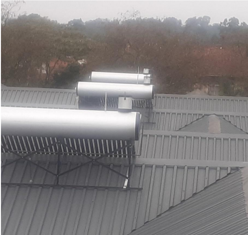
Aggluton, Harare 7x300L Direct Thermosiphon systems individually mounted on each housing unit
