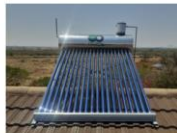
Figure 2. Thermosyphon system (CPS Sisters Convent of Lady Kingsdale) - view from north, December 1987
