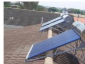
Figure 1. Thermosyphon system (CPS Sisters Convent of Lady Kingsdale) - view from north, December 1987
