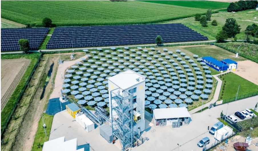
Solar tower with reactor for fuel production at 1,500 °C in Germany, demonstrator by startup Synhelion, Switzerland Photo: Synhelion
